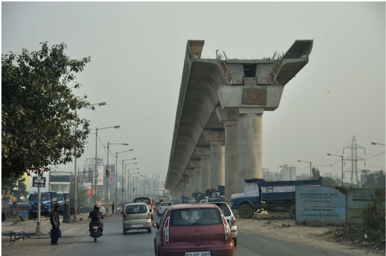
An elevated railway under construction in Kolkata. 15
