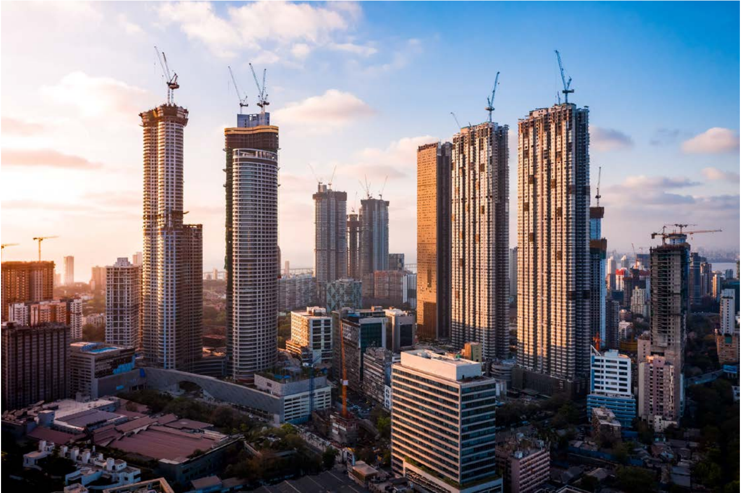
Skyscrapers under construction in Mumbai. 1
