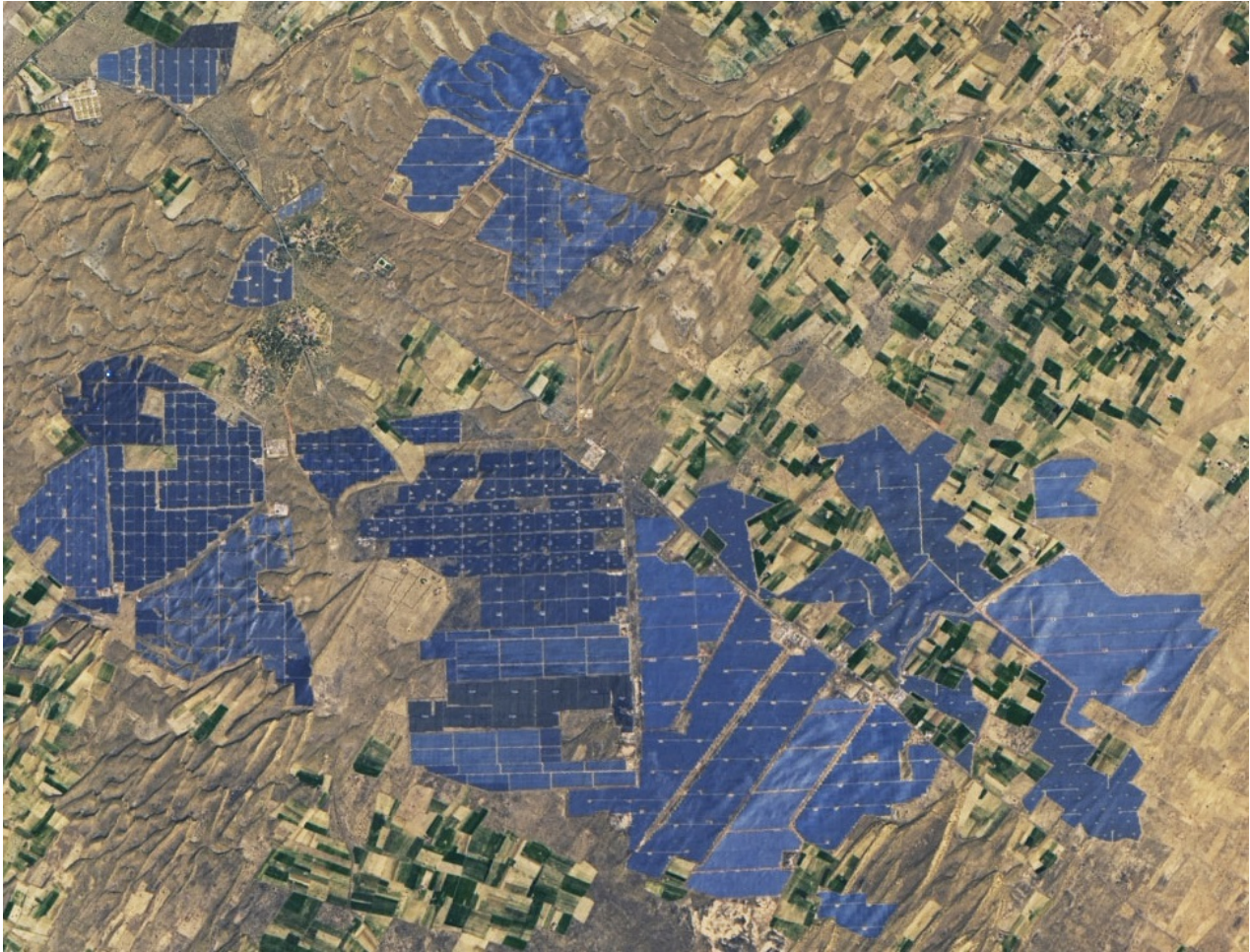
Satellite view of Rajasthan's Bhadla Solar Park, the largest solar farm in the world. 46
